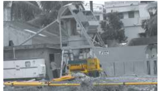
BP 350 pumping concrete with CP 18 batching plant
